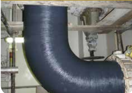
Pipe repair & reinforcement
